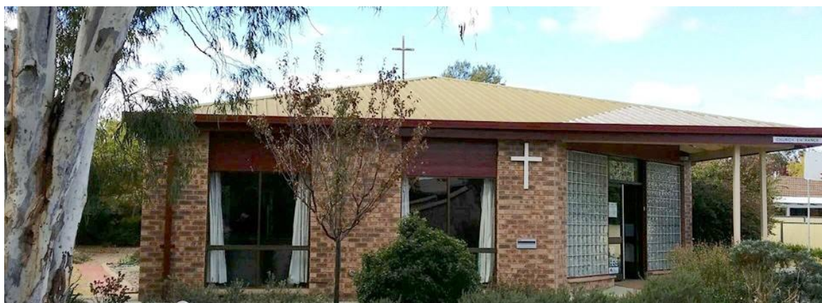
Figure 1: St Simon's Anglican Church, front entrance
