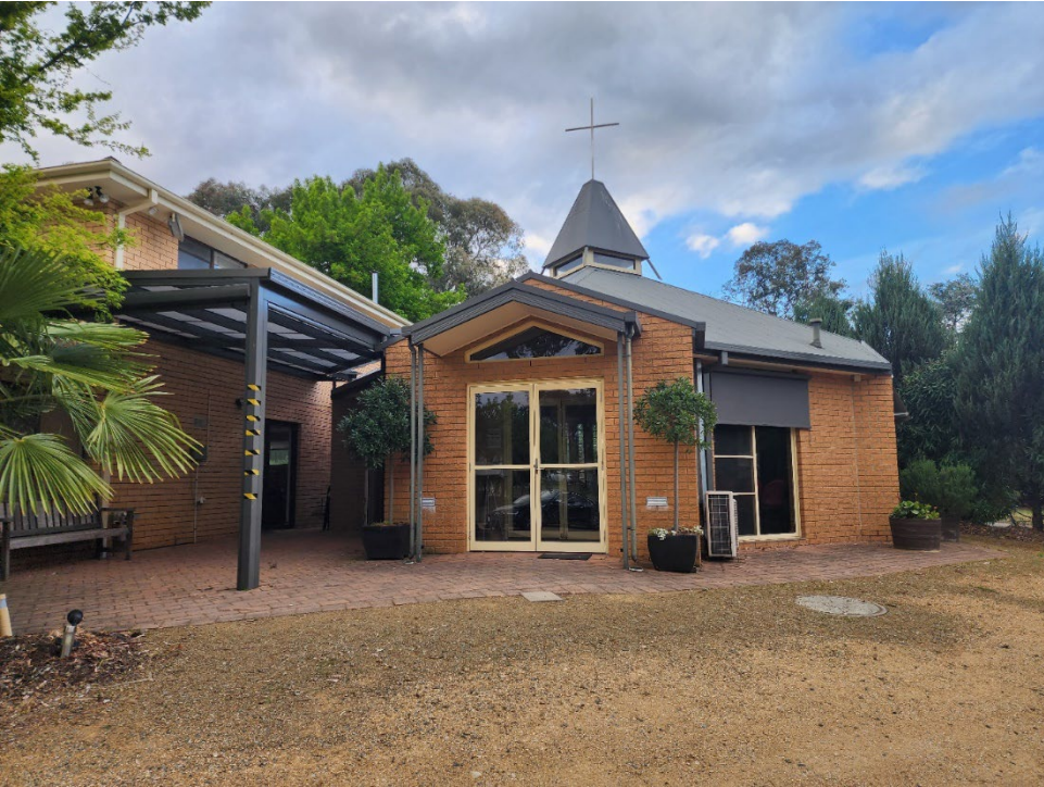
Front view of church
