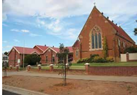
St Luke's Anglican Church June [68]. Photo provided by St Luke's
